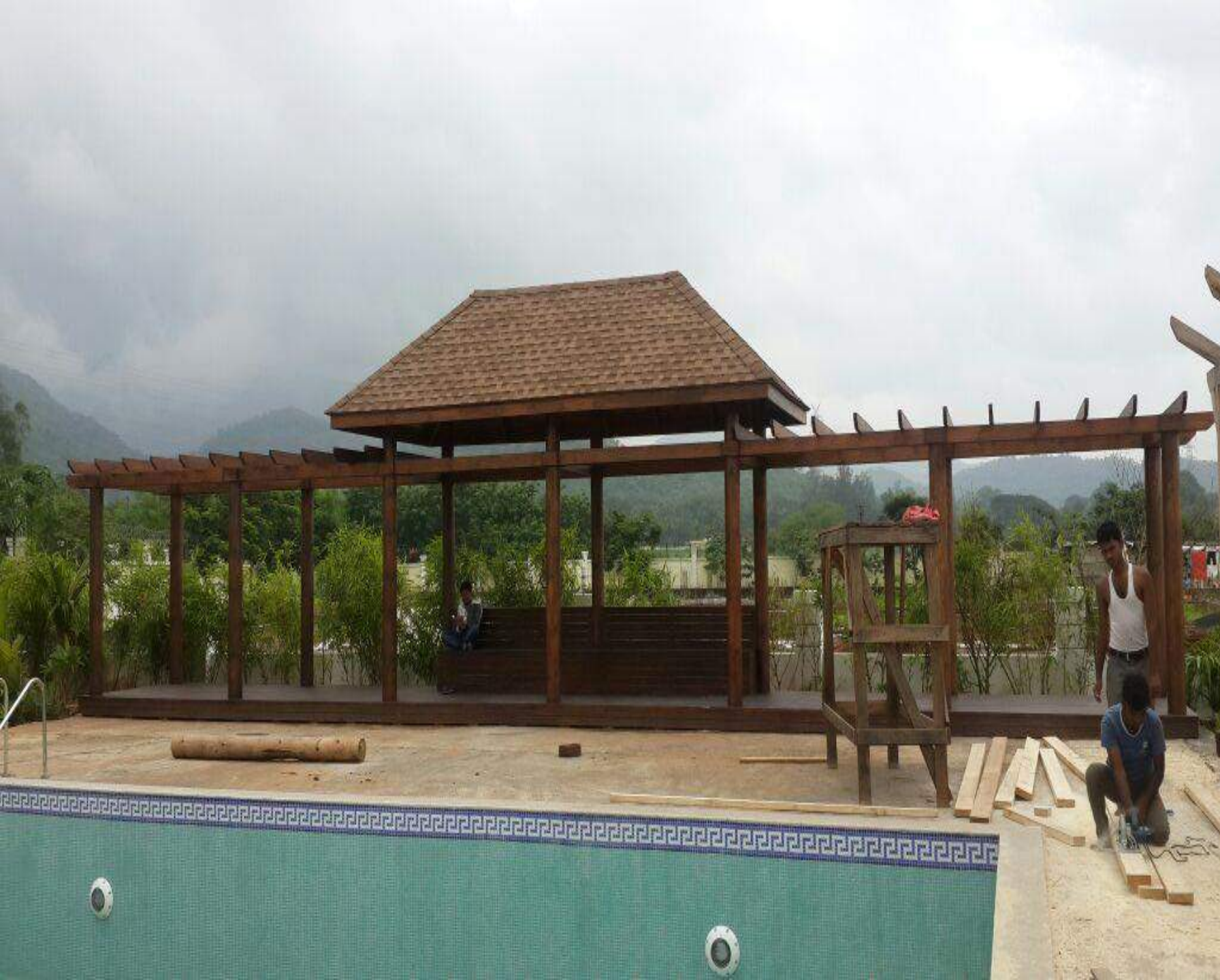
Mumbai, Gazebo near Swimming Pool
